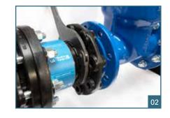
Hook the hook wrench into one of the grooves on the loose flange side of the QUICK-TWIST as shown.
